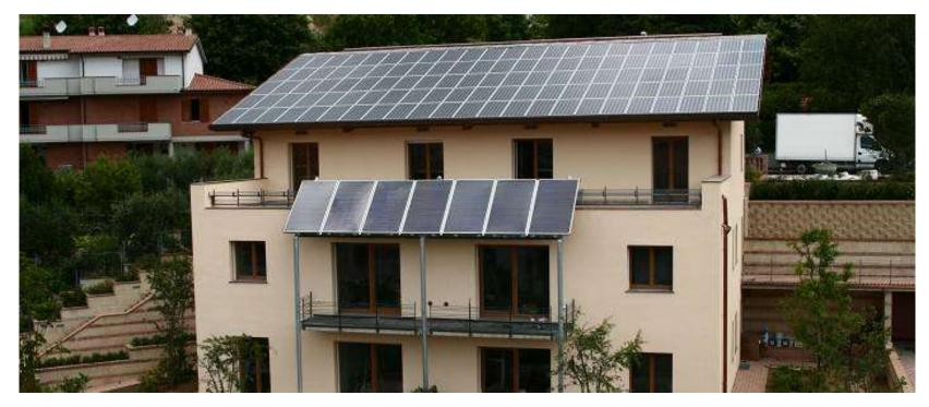
The LH has a grid-connected PV system (20 kW nominal power) composed of 115 panels. The system covers the entire roof surface (150m²), facing the south. The panels are arranged in nine strings and are connected to three inverters. The nominal declared efficiency of the PV panels is 12%.
